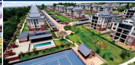
Crowthorne Luxury Apartments Located on Whisken Rd, Midrand, Joburg
