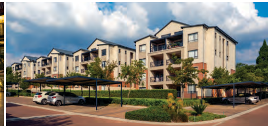
Crowthorne Luxury Apartments Located on Whisken Ave, Midrand
